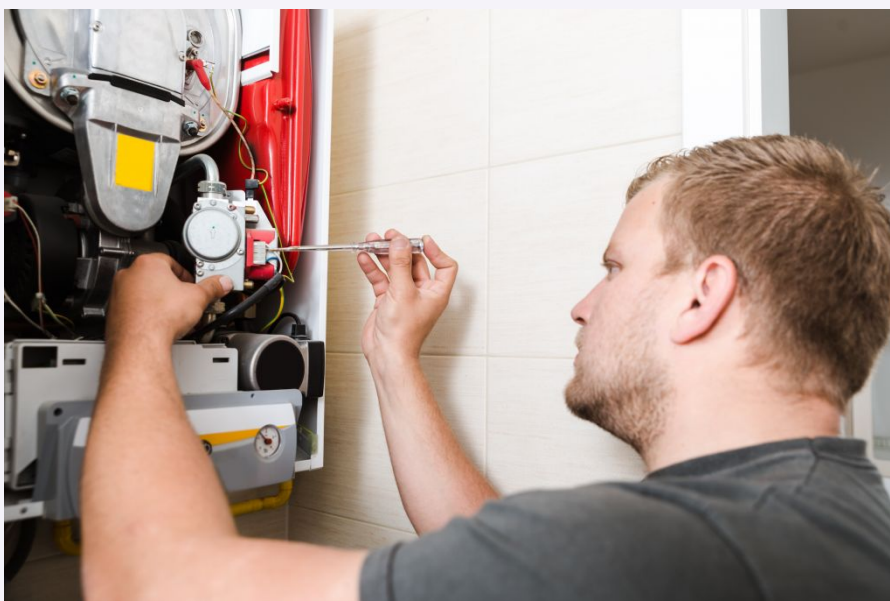
Figure 7. A technician performing a repair on a central heating boiler.
